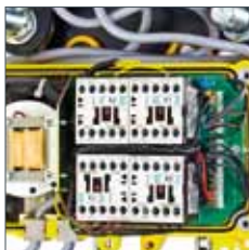
Increased operating safety through 42 V control voltage
